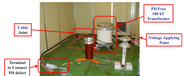
Fig. 4. The XLPE cable with a PD free 100 KV Transformer
